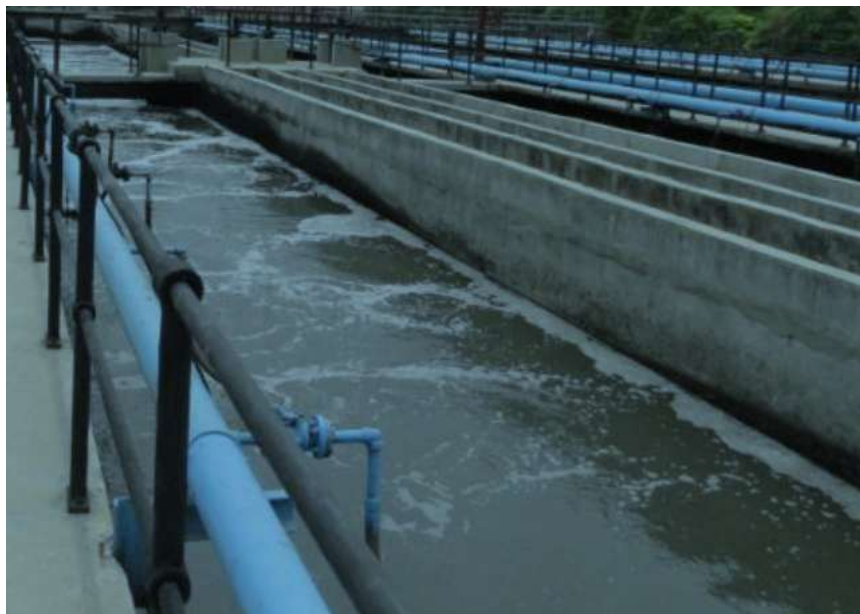
Figure 9 Aeration tank
