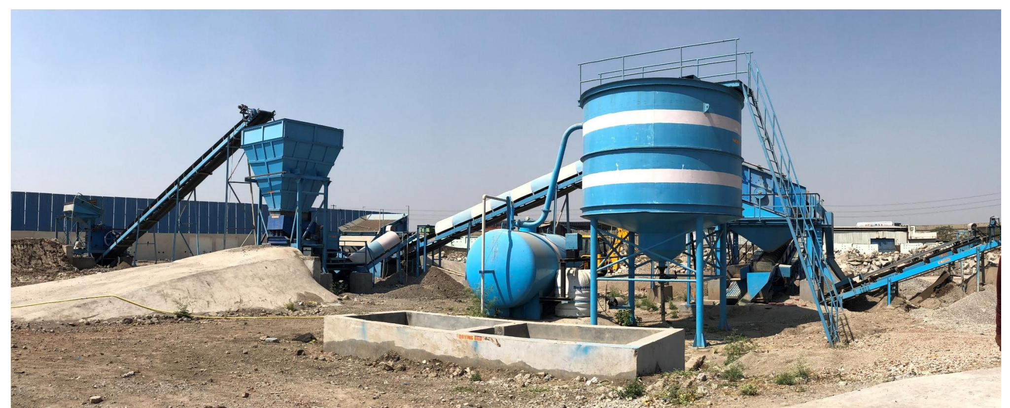
Construction and demolition waste treatment plant
