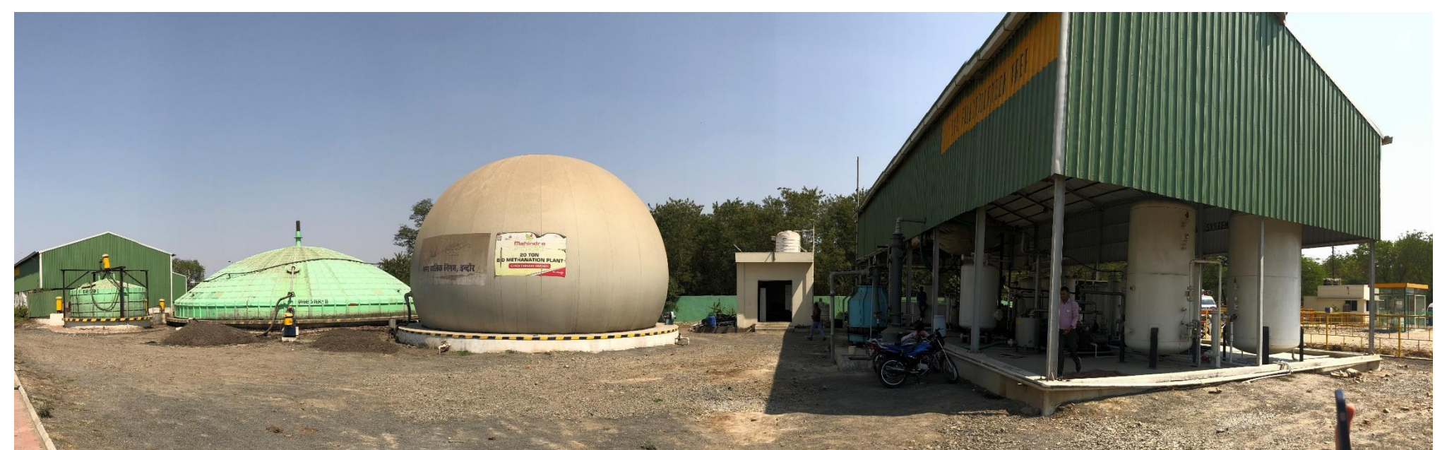
Bio-methanation plant practising conversion of wet waste from bulk generators into biogas
