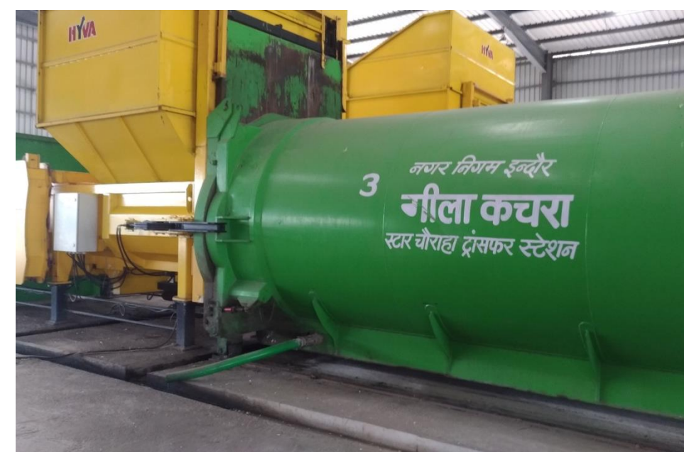
There are two separate hoppers for dry waste (Blue colour) and wet waste (Green). The segregated MSW is compressed into respective containers
