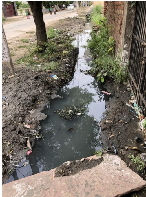
Figure 24: Chocked drains in Sohna MC area
