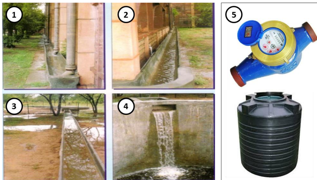
Figure 54: Rooftop rainwater harvesting installed at Central Arid Research Institute, Jodhpur (Subfigures 1-4). Smart water meter and tank (Subfigure 5) [Courtesy: Google images]
