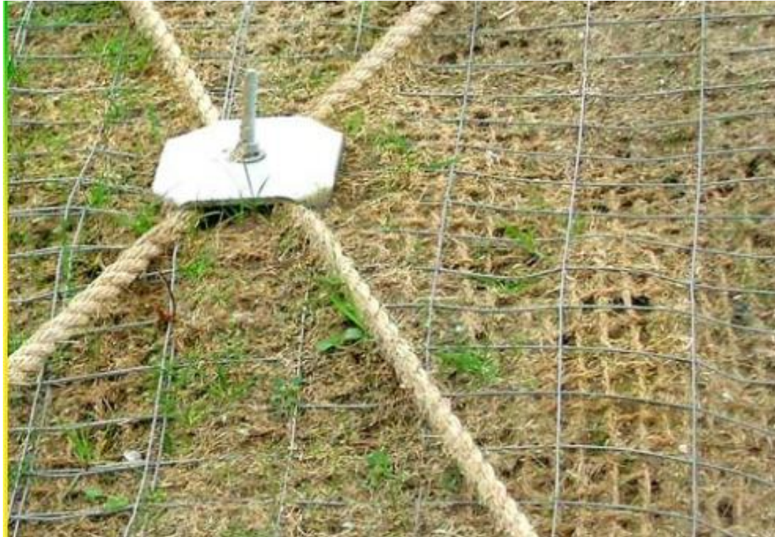
Figure 41: Wire net over coir mats 14
